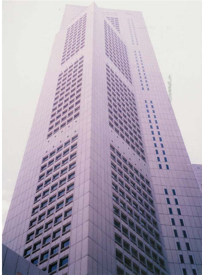
Overseas Union Bank Building, Downtown Singapore
