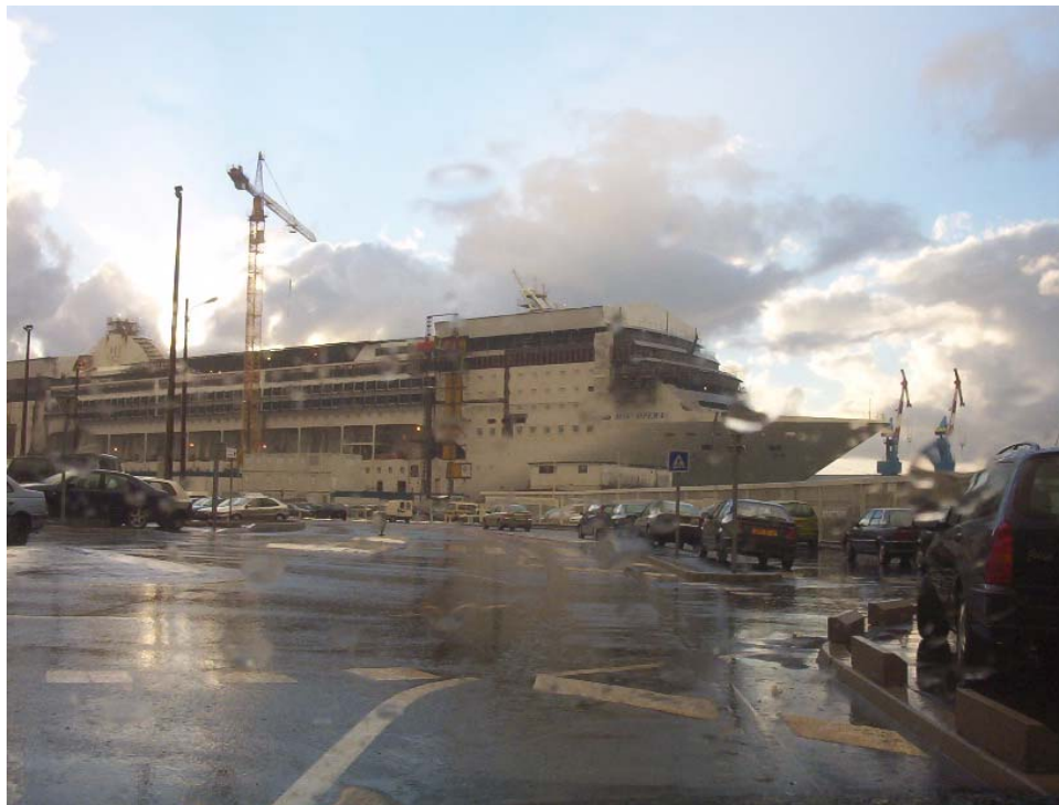
Opera under construction at Saint-Nazaire
