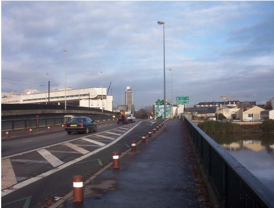
General Audibert Bridge (Eastern Span, Western Span slightly higher)
