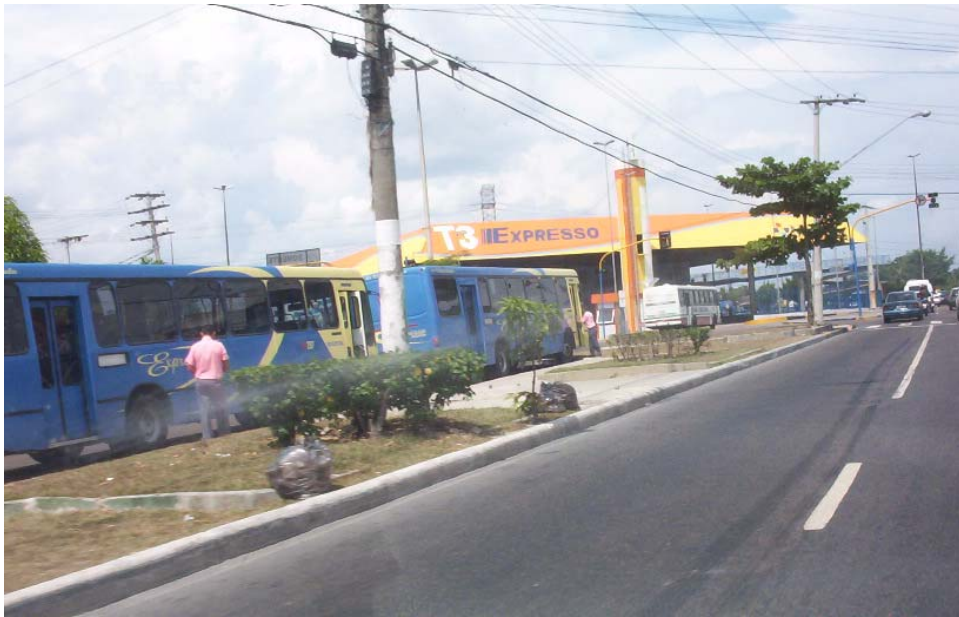
Busway and Bus Terminal (Transfer Station)
