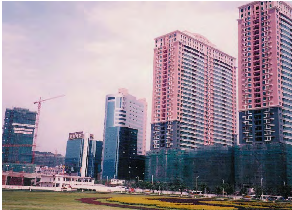
Commercial and Residential Buildings
